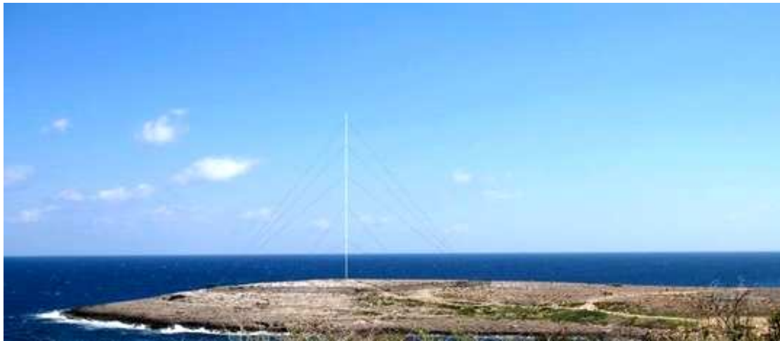
The 80-metre mast to analyse the Sikka I-Bajda off-shore potential
